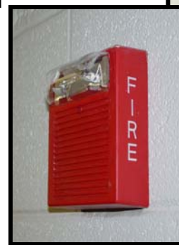
Fire Alarm Horn/Strobe
